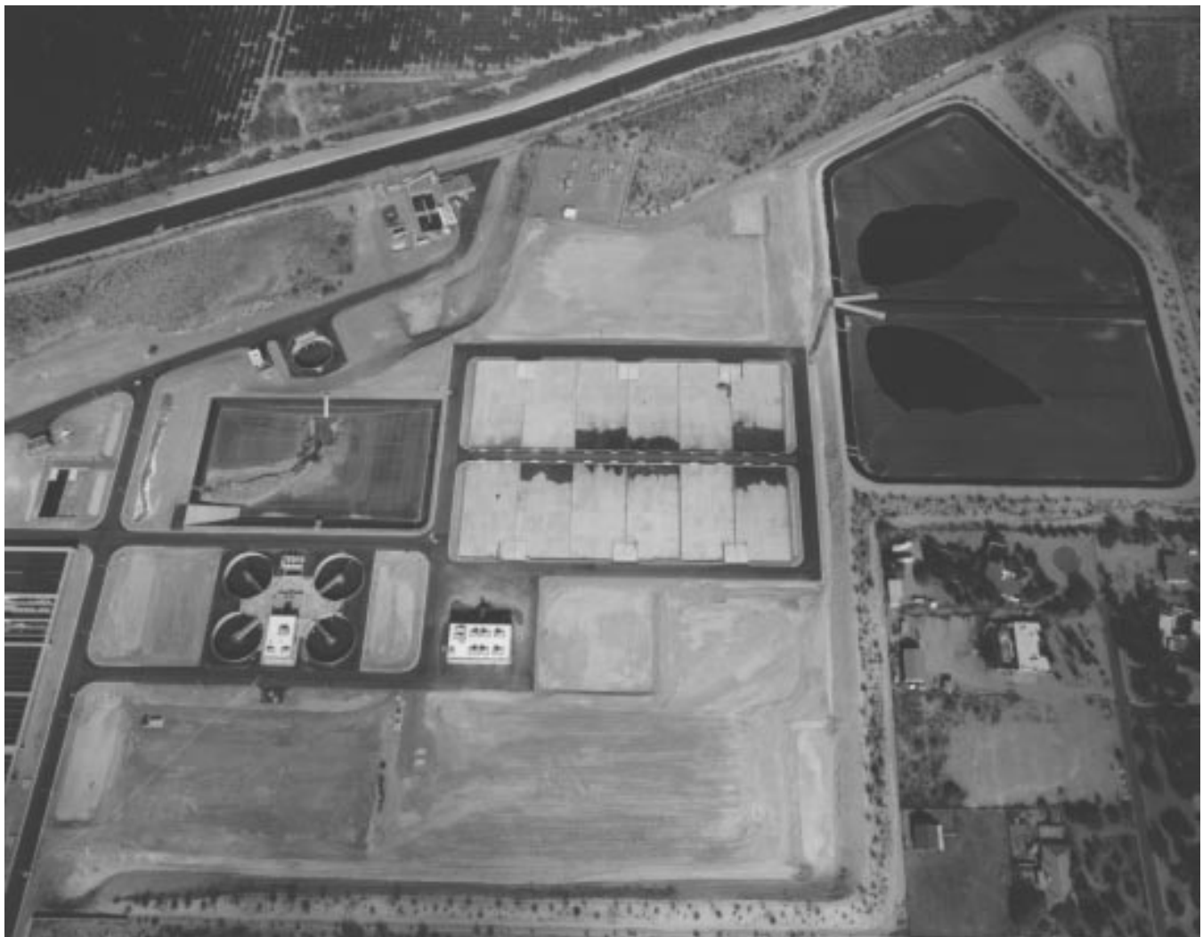
Figure 4-17. Aerial view of residuals handling process system, Val Vista WTP, Cities of Phoenix/Mesa, AZ (John Carollo Engineers, 1994).
